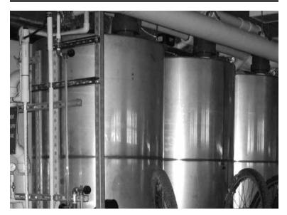
The rainwater collection system at our Riverside Park branch (see the cisterns above) covers ½ of our toilet flushing needs. Using rainwater helps us conserve 100,000 gallons of clean, filtered water per year.
